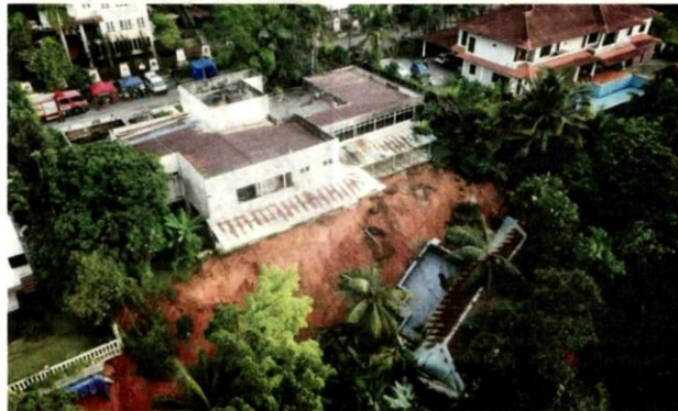
KEADAAN tanah runtuh di Kemensah Heights.
