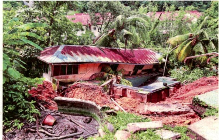
One of the houses affected by the landslide in Kemensah Heights, Selangor, on Friday. PIC BY FATHIL ASRI
